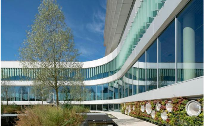
Front view of the city hall showcasing its green façade and interior gardens. The constructed wetland filters and recycles water, including rainwater and sink water, for use in the green façade and flushing toilets (Source: Ronald Tilleman from <u>The Plan website</u>)
