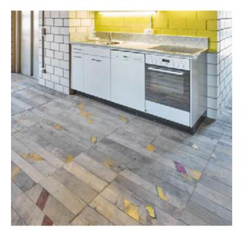
Interior image that shows the granite slabs from the Orion office façade repurposed as kitchen floors (Source: Martin Zeller).
