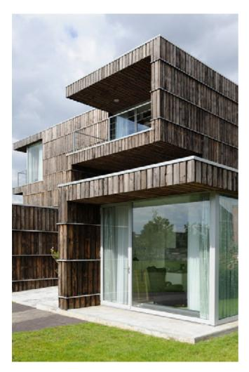
The façade of the building was constructed using cable reel slats (Source: <u>Superuse Studios</u>)
