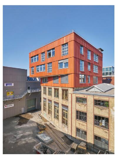
Overview of the K.118 building exterior, showing the contrast between the original building and the additional floors following the renovation and expansion (Source: Martin Zeller).
