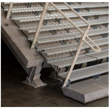
Images showing the concrete slabs from the original floors being cut and tilted to fit new stairways (Source: Hampus Berndtson)
