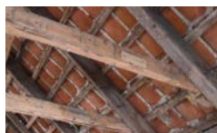
Roof tiles Aggregate
