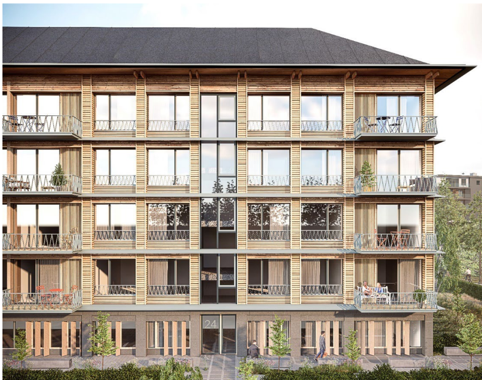
Figur 71 Biogen renovering – nyrenoveret
