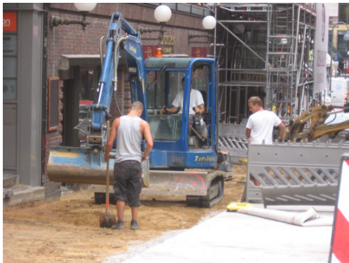
The new design under construction: BID Hohe Bleichen (all photo: Schote)
